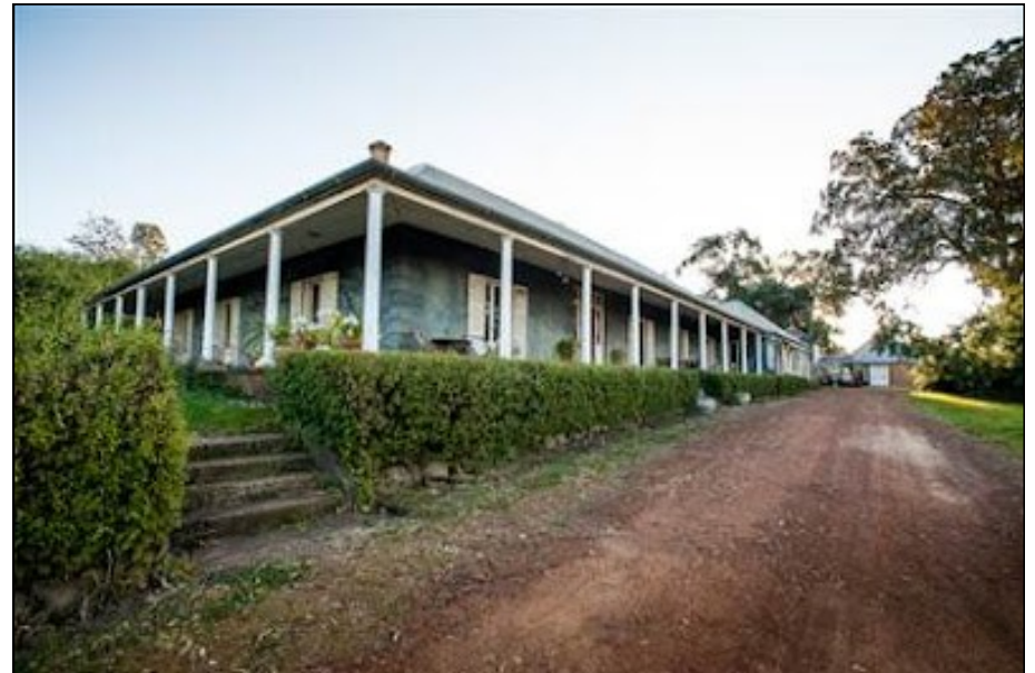
Maryland House c.1990s (rs.locationshub.com)
