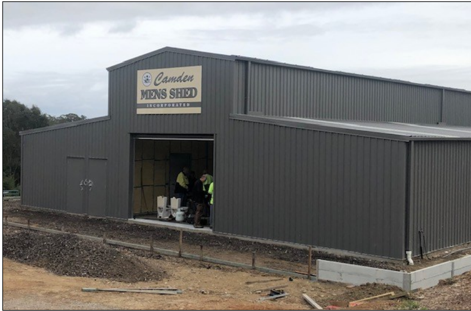
Camden Men's Shed (W Sims)
